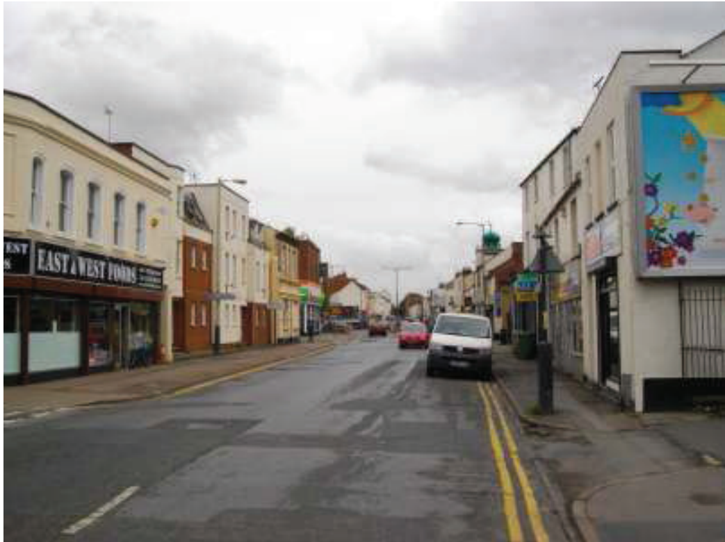
Site 3. High Street towards Tewkesbury Road junction (view east)
